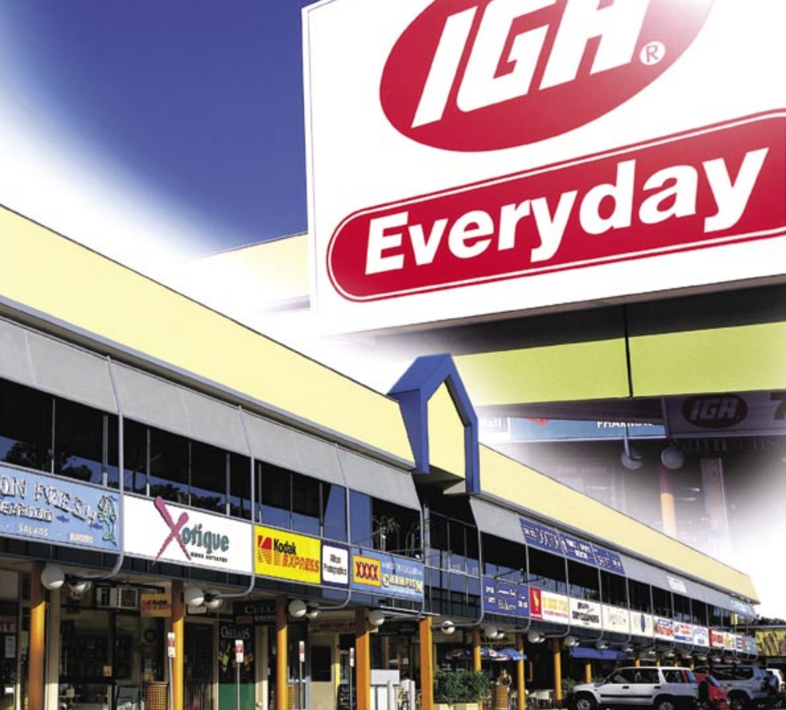
Milton Village Shopping Centre, Milton, Queensland
