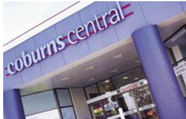
Coburns Central Shopping Centre, Melton, Victoria
