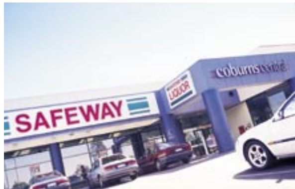
Coburns Central Shopping Centre, Melton, Victoria
