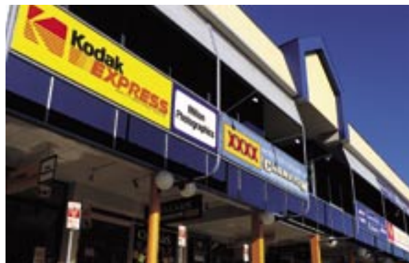
Milton Village Shopping Centre, Milton, Queensland
